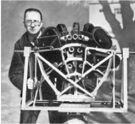
◀ Fred Waller with the 11-camera Vitarama set up created for 1939 World Fair. Cinerama's three-projector set up lead to some dramatic film (right)
